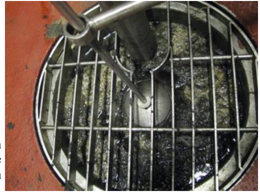
Here is a drain at a corn factory, again notice the black scum
