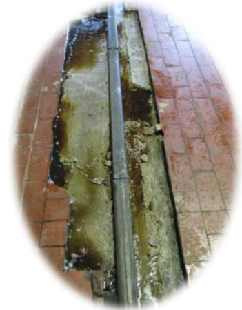
This is in a receiving dock, notice the oil in the rail car lines, black scum and gassing evidence
