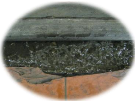
This is in a receiving dock, notice the oil in the rail car lines, black scum and gassing evidence
