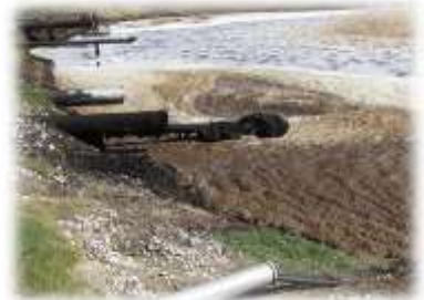
Aerobic lagoon at a coffee plant
