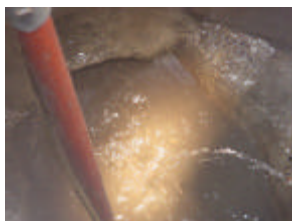
Sewer slime from metal cutting plant- many oils used in cutting steel parts
