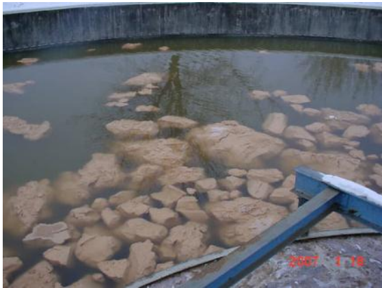
Zooglea is also very hard to dewater, and adds significant weight to your solids. Polymers cannot help Zooglea, and adding chlorine to your aeration basins with Zooglea will only make it worse.
